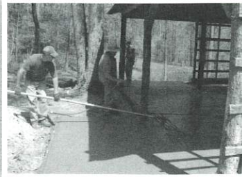
Pouring cement floor for Farm Barn.
