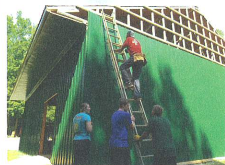
Wake Chapel hung all of the metal siding and soffits on our new Maintenance pole barn and helped move stuff from the Work Shop into the new pole barn.
