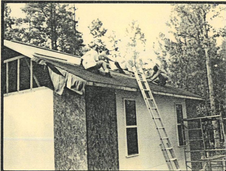
Larry, Shawn, Kevin & Todd shingling the roof of the office.
