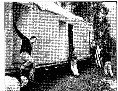
All of the nails and staples have to be removed from the wall that joins the two halves of the modular. Missionary Ann Sampson, her husband Doug, work along side Larry and other volunteers.
