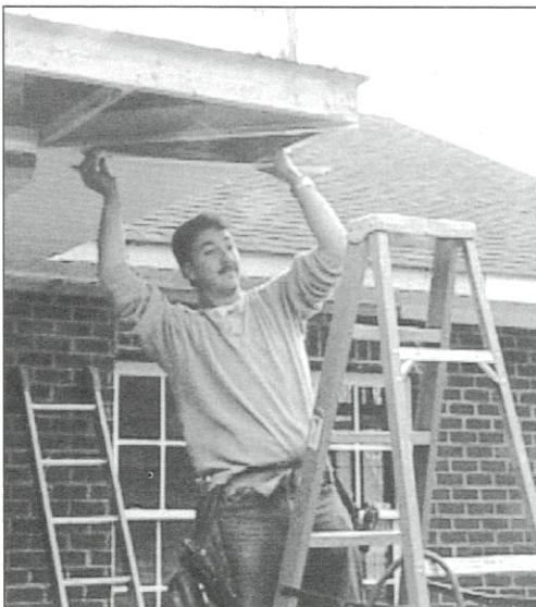
Steve Wooten works to put up the soffit on the exterior of the building.
