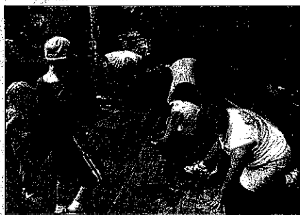
Putting brick pavers in place for the new sidewalk to the Prayer Rock.
